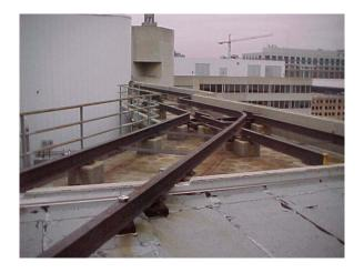
Comment: Removal and replacement of 31,000 SF of Modified Bitumen Membrane with a new insulated, torched down Modified Bitumen Roof Assembly . Work included removal of a structural steel window washing track, repairs to precast parapet panels and repairs to the precast wall panels.
